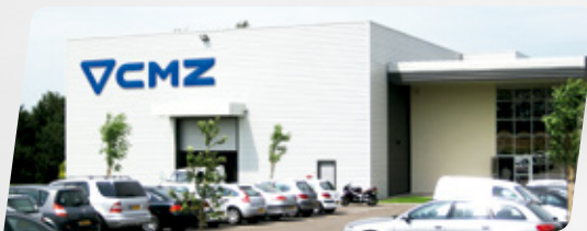
HANDELSBÜRO | AFTER SALES SUPPORT SERVICE | SHOWROOM Vaulx Milieu – France
