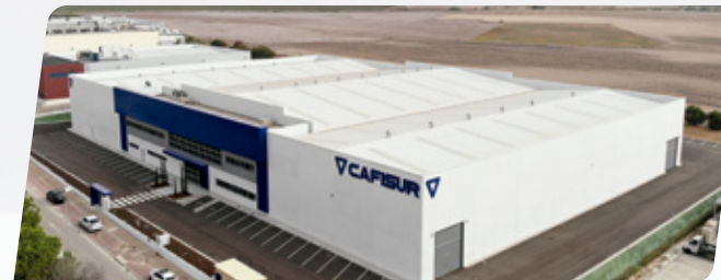
Sheet metal plant 15,000 m2 | Cádiz – Spain
