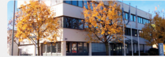
CMZ Deutschland HANDELSBÜRO | AFTER SALES SUPPORT SERVICE Stuttgart – Germany
